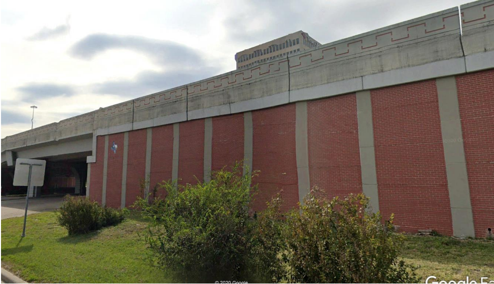
MSE Retaining Wall: IH 610 @ Bissonnet St (Houston)
