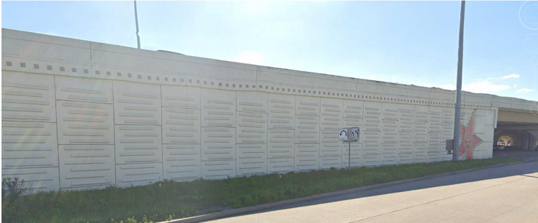
MSE Retaining Wall: I-10 @ Katy Fort Bend Rd (Katy)
